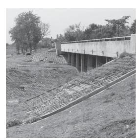
left. Embankment, right. Stabilised embankment and culvert to prevent gullying
