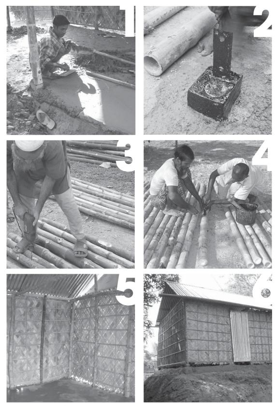
Building a flood-proofed house: 1. Cement stablised earthen plinth, 2. Concrete stumps to hold bamboo posts off the ground, 3 and 4. Treating bamboo against insect infestation, 5. Walls and floor of house, 6. Raised house. (UNDP Flood Recovery Programme in Bangladesh)
